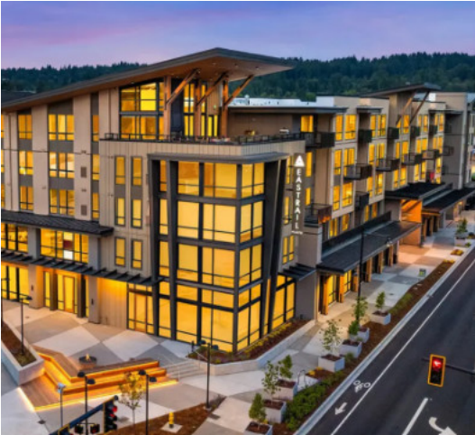
Figure 31 -Roof Form Varied roof form with fully integrated roof overhangs and parapets.
