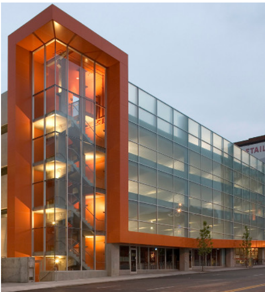
Figure 129 - Parking Garage Screening
