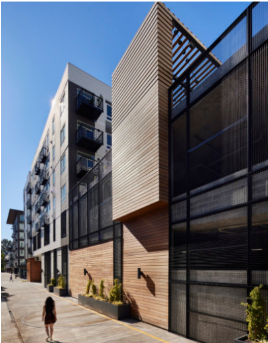
Figure 40 -Service / Loading Screening Alley Side Screening integrated with the facade design and landscaping.
