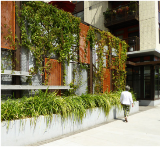
Figure 128 - Parking Garage Screening
