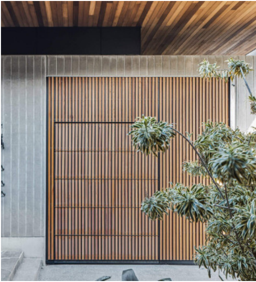
Figure 39 -Service / Loading Screening Slatted wood screen at service/loading area
