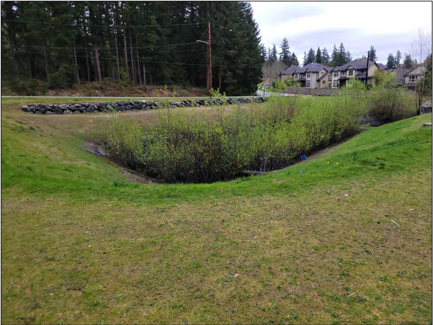
WSDOT stormwater pond looking generally southeast. Note rockery wall adjacent to North Creek Drive and young trees in bottom of pond.
