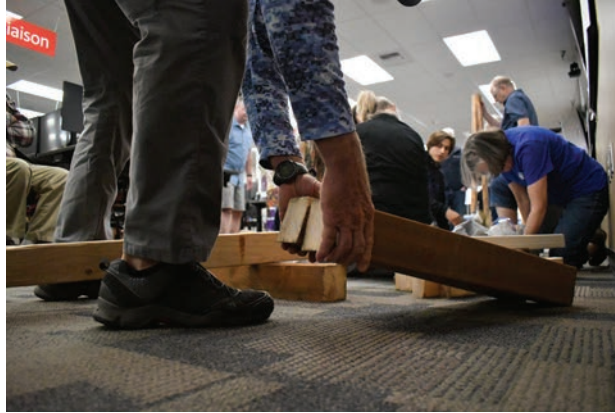
Students practice cribbing to lift a simulated collapsed structure, and improvised tools to bust through walls, including just a pencil.
